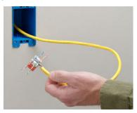
Step 3: Insert jack in JackRapid front first with IDC slots facing blades of JackRapid.
