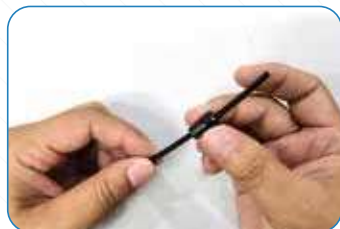
2.1 Put the cable into the boot
